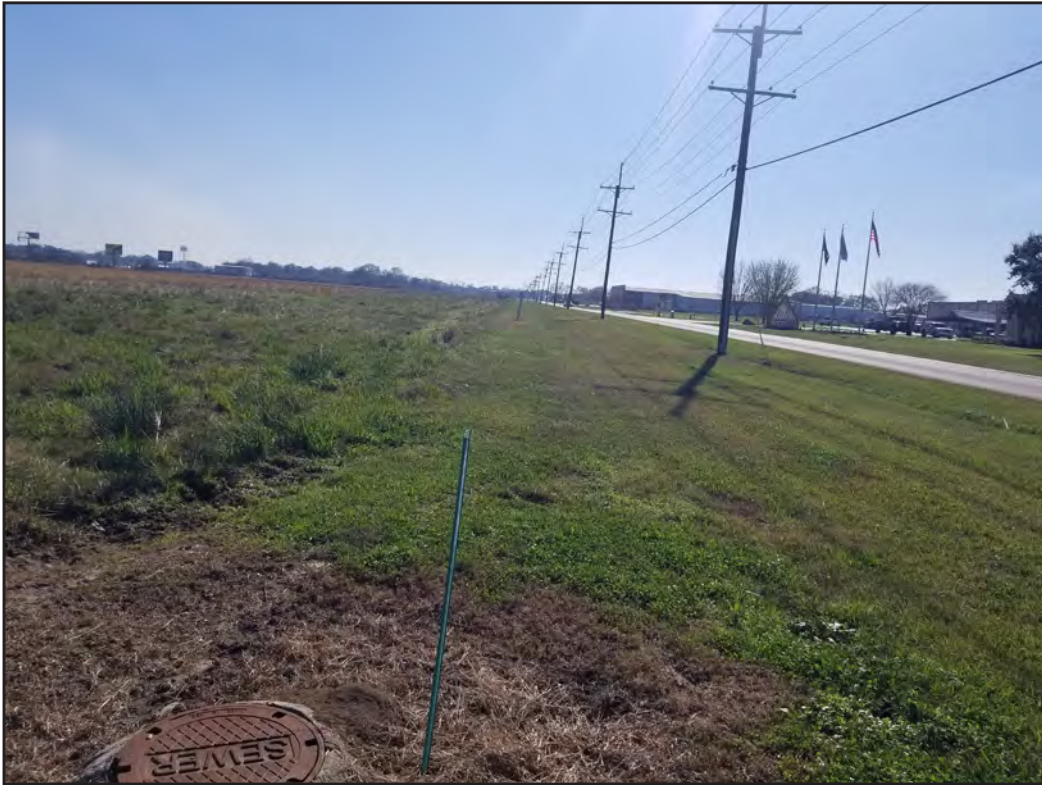
Figure 5.5. View of the transmission and sewer line easements on the west side, facing south.
