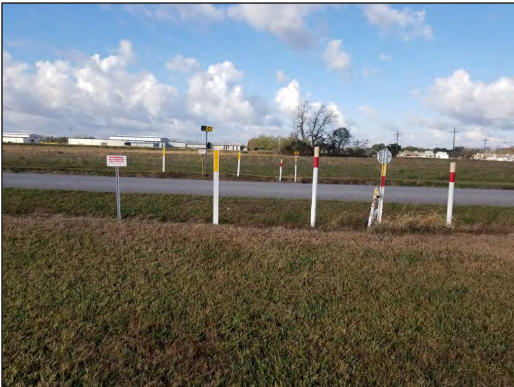
Figure 5.6. View of natural gas and petroleum pipelines crossing the project area, facing west.
