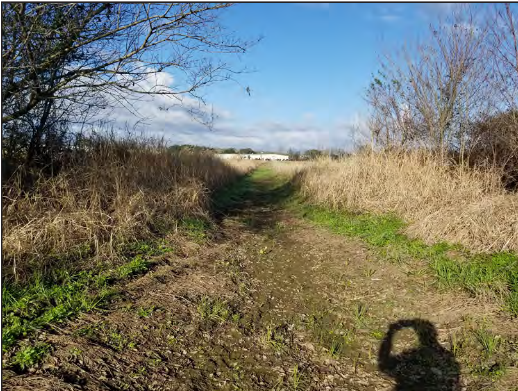
Figure 5.9. View of the southernmost earthen canal, facing west.
