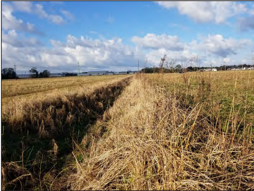
Figure 5.7. View of the northernmost earthen canal, facing west.
