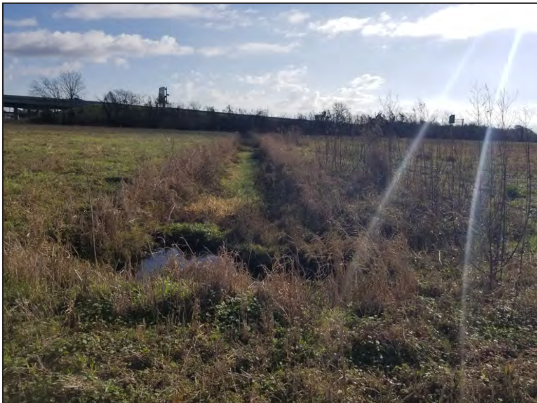
Figure 5.8. View of the central earthen canal facing east.
