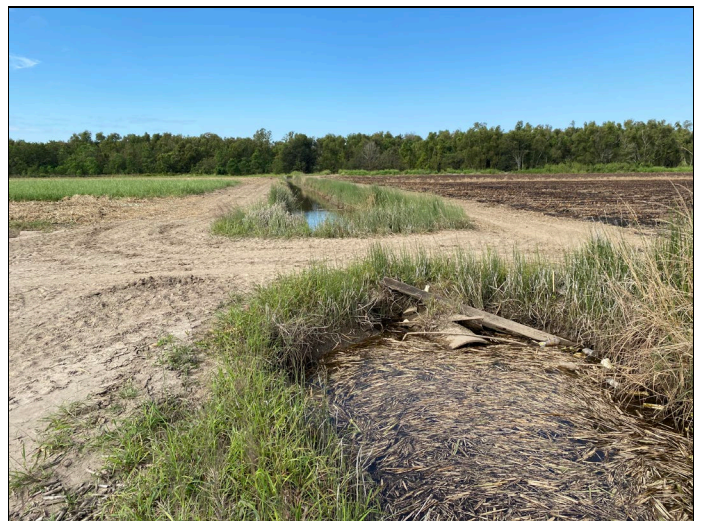
12. Drainage ditches in the northwest corner of the property
