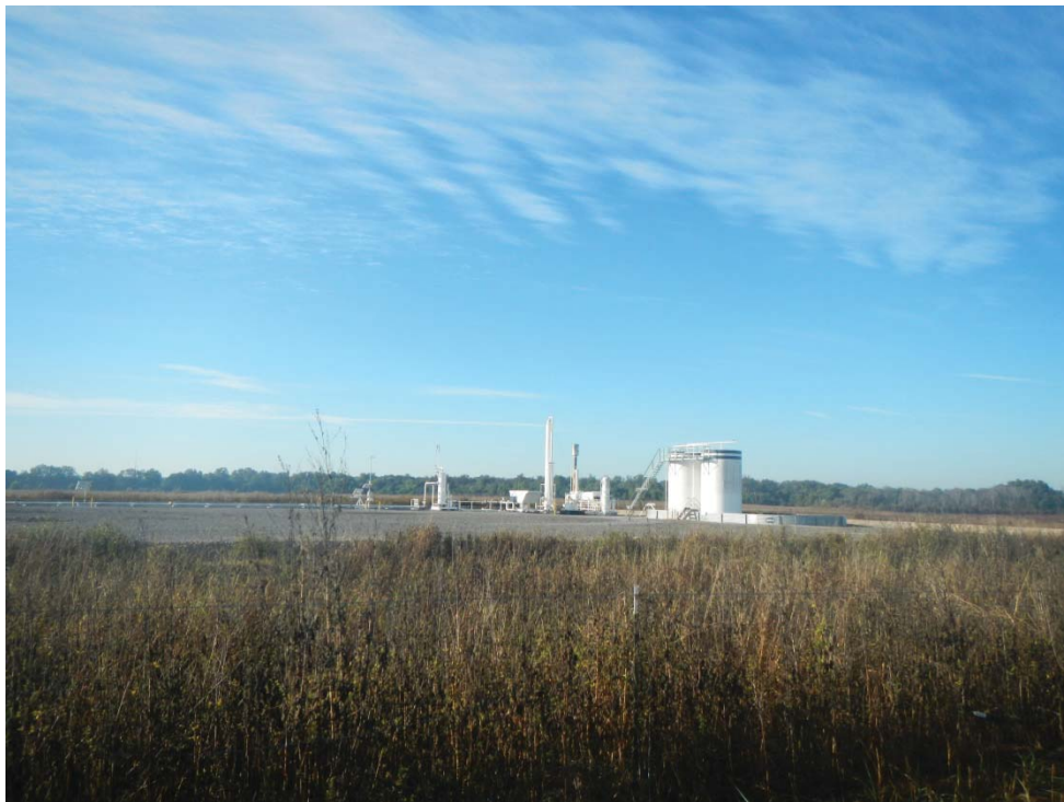
Chesapeake Operating, Inc. well site located near the north-central portion of the assessment property.
