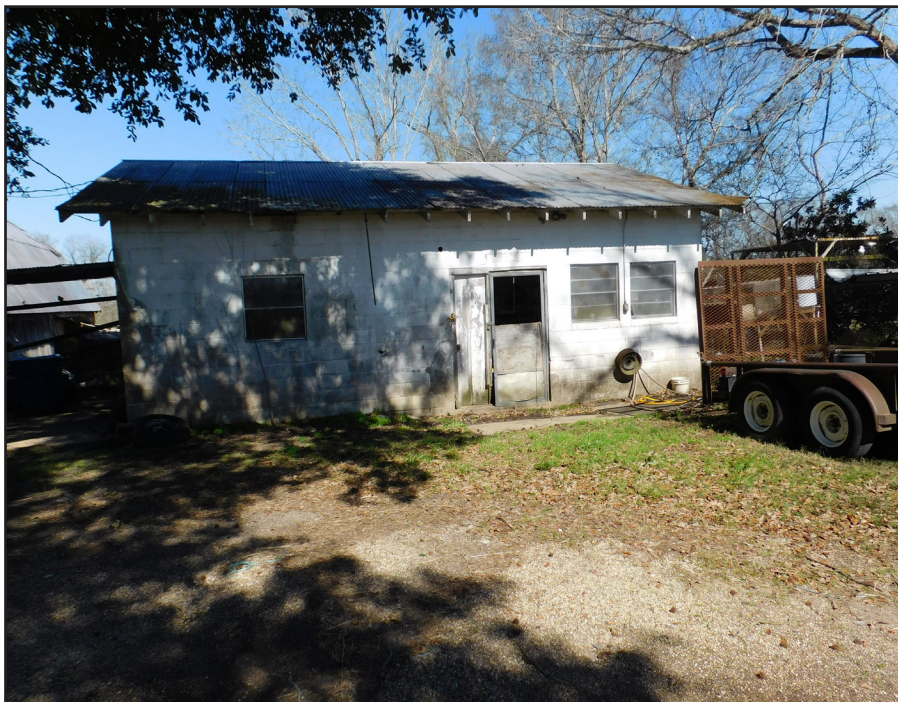
Figure 5.16. The south façade of Resource 1c, facing north.
