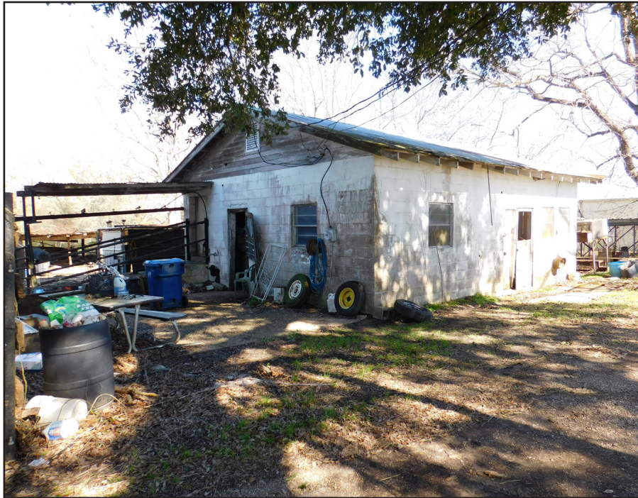
Figure 5.17. The southwest oblique of Resource 1c, facing northeast.
