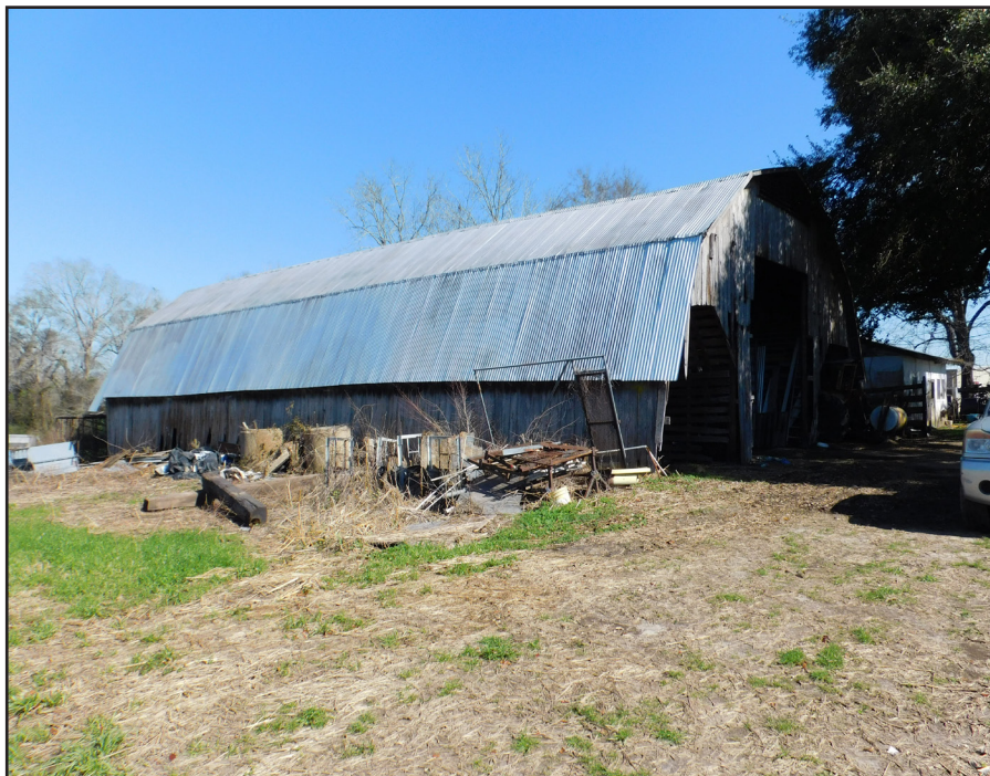
Figure 5.14. The west façade of Resource 1b, facing east.
