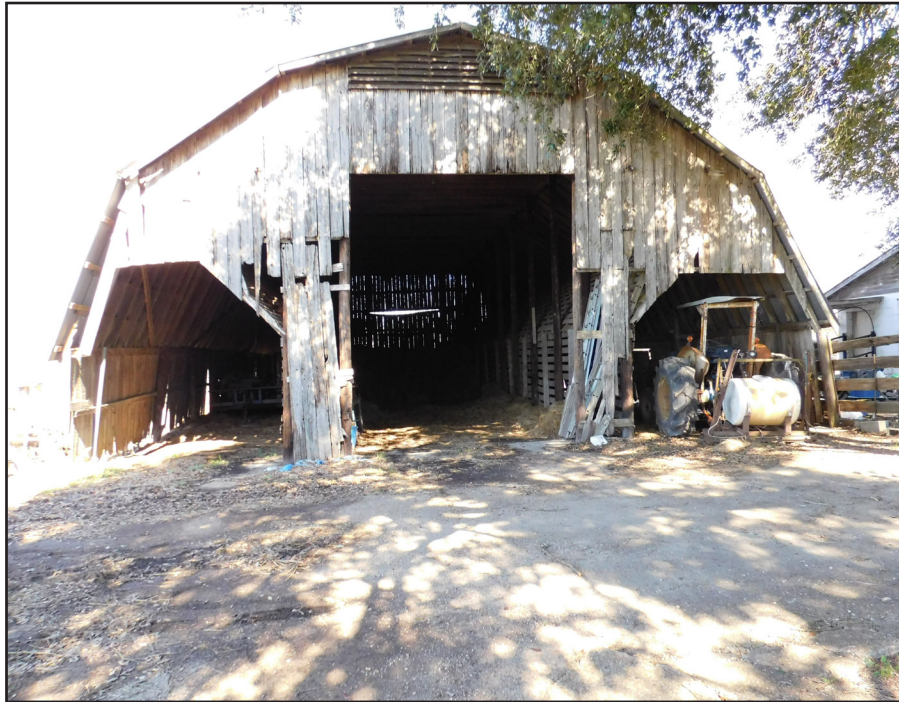
Figure 5.13. The south façade of Resource 1b, facing north.
