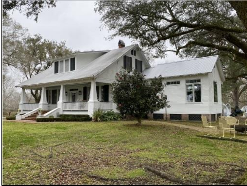
Figure 30. Exterior view of Structure 50-00789.
