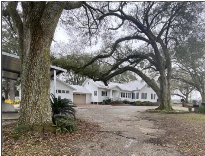
Figure 31. Exterior view of Structure 50-00789.
