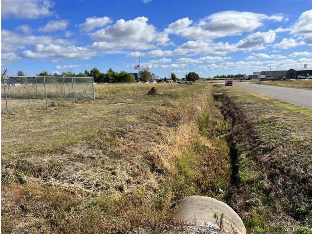
Figure B.23 View looking to the east from southwest property corner showing the roadside drainage ditch along southern boundary - (CEI 11-07-23).
