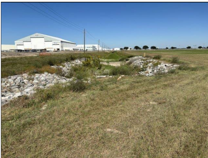
11. Drainage ditch north of the site
