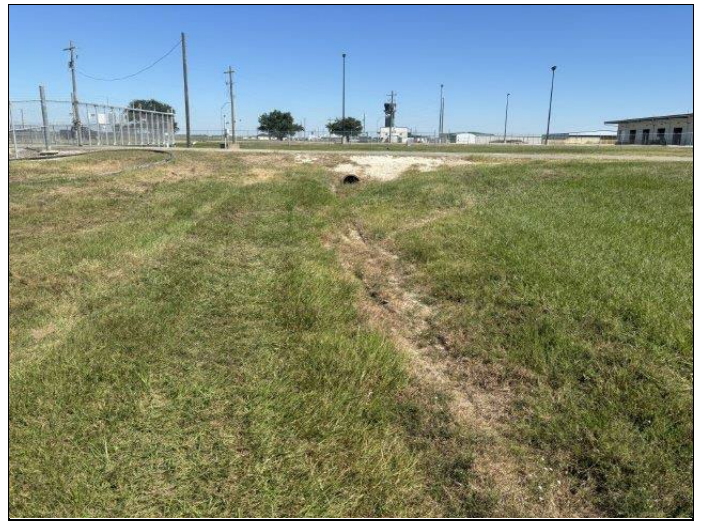
8. Ephemeral drainage swale
