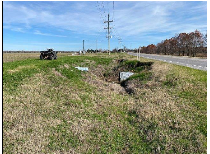
4. Drain pipe and culvert that flows beneath LA 131 to Whitehall Lake
