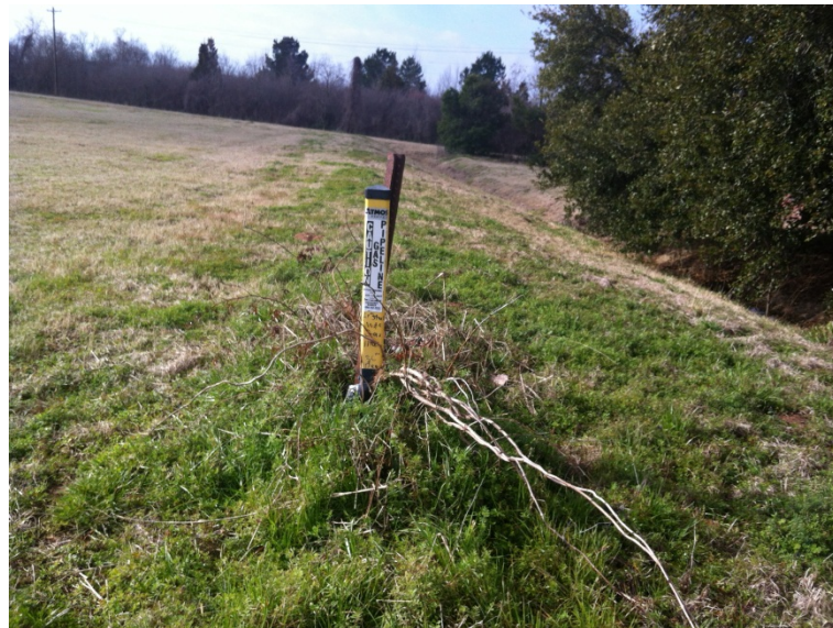
Gas Pipeline Marker on West Edge of Property
