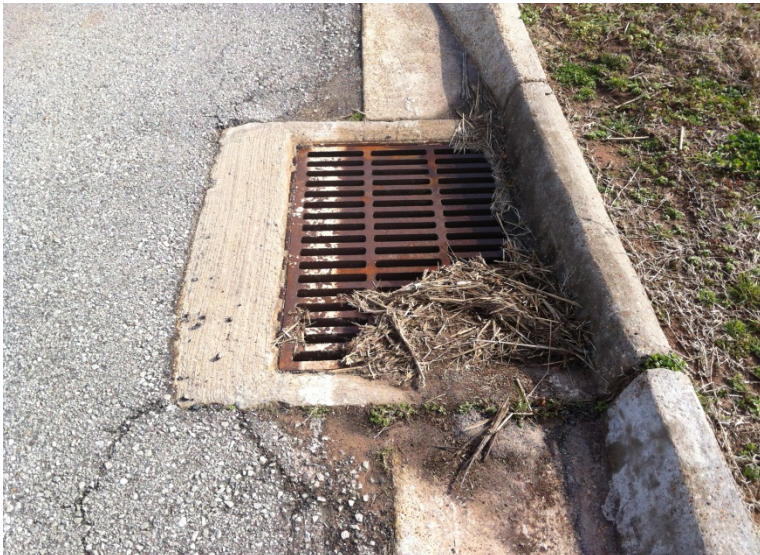
Storm Drainage on Industrial Drive
