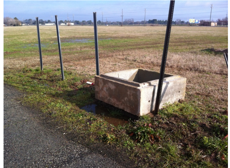
Used Square Concrete Culvert
