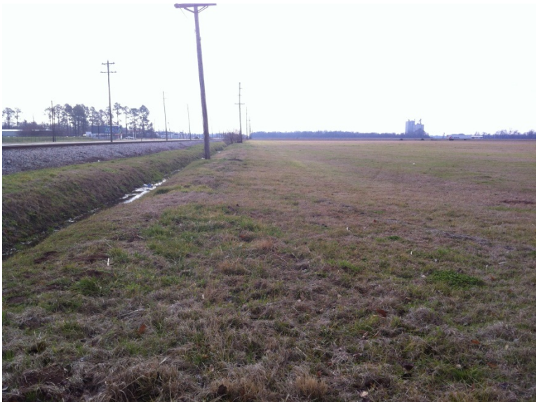
Drainage Ditch and Railroad Tracks, facing East
