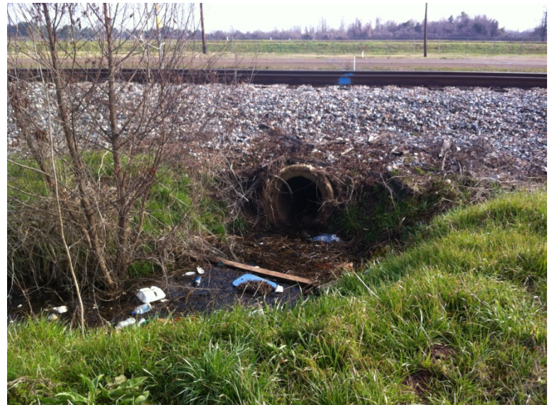
Drainage Culvert Under KCS Railroad Tracks
