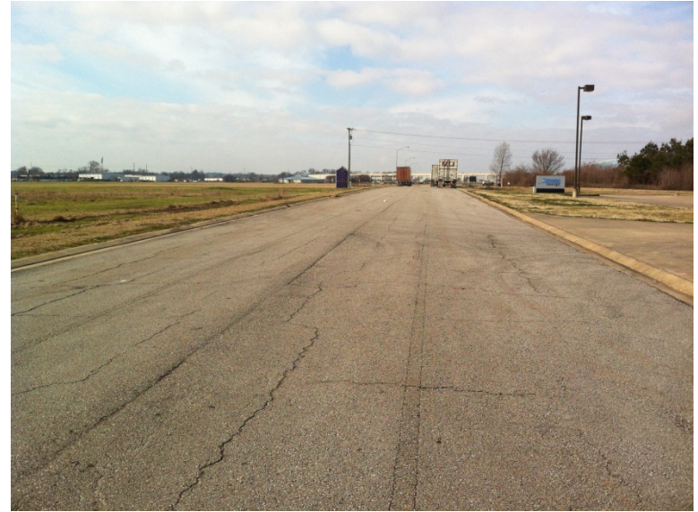
Industrial Drive, facing South
