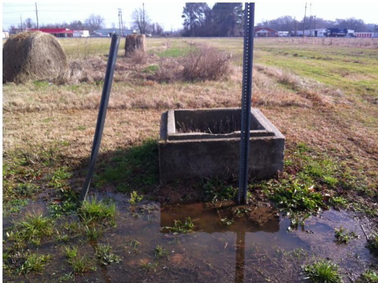
Used Square Concrete Culvert
