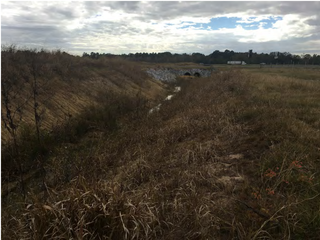
Photograph 12 View of Drain along Eastern Property Line Facing South
