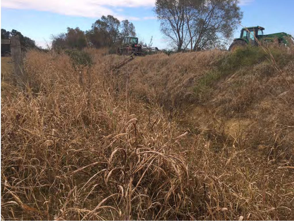
Photograph 11 View of Drain along Eastern Property Line Facing North
