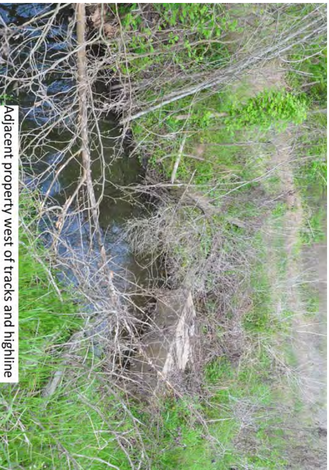
Debris along railroad tracks
