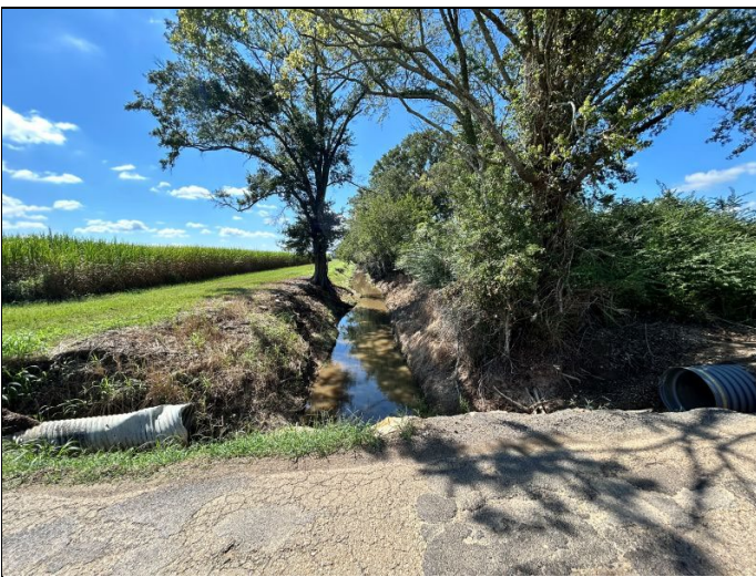
11. S3 – Drainage canal on eastern boundary
