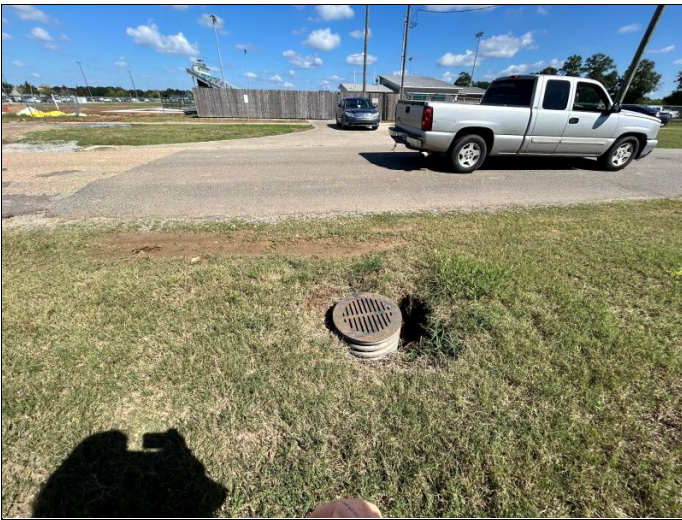
9. S2 – subsurface drainage pipe on northern boundary
