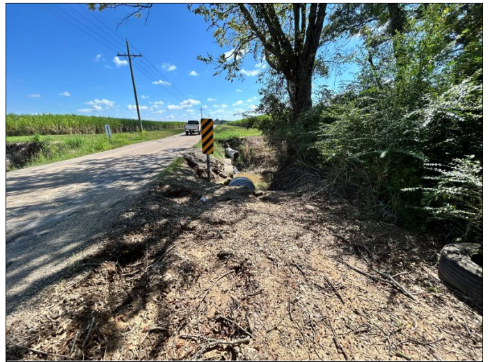
10. S2 – outfall into S3
