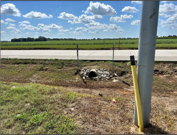
13. S1 connection to southern property
