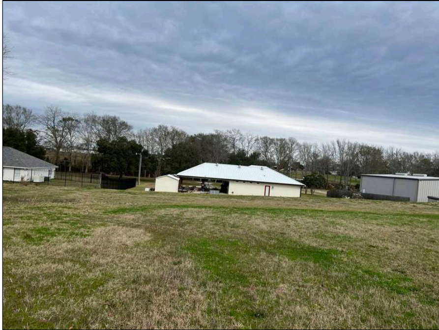
29 - Photo 29 : Overview at PP3 facing north.
