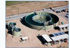
The completed plant is filled and commissioned.
