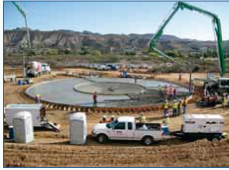
The foundation is prepared and rebar is installed based on foundation plans provided by Ashbrook Simon-Hartley. A working supervisor is also provided to assist with embedded item placement, and to witness the pour.
