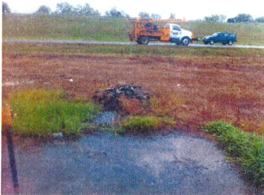
Description: Stressed vegetation and small area of debris near concrete slab.
