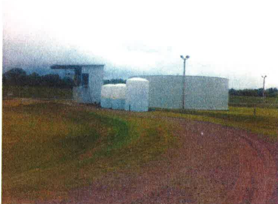
Description: Fertilizer storage tanks south of subject property.
