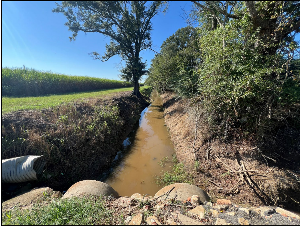
Photograph #9 NE corner of Subject property looking south, drainage canal visible.
