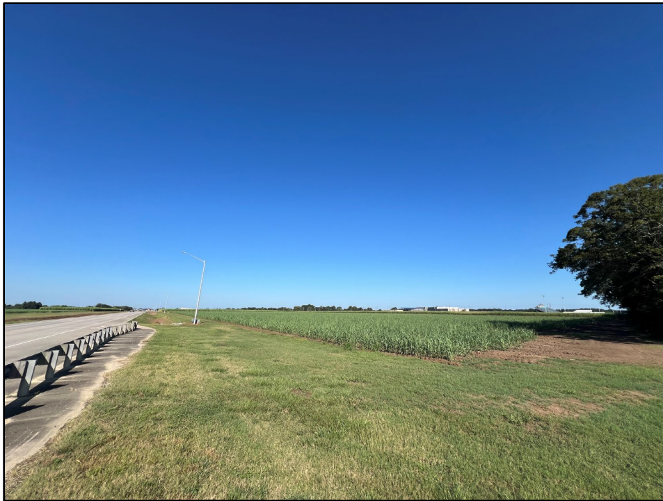
Photograph #11. SE corner of Subject property looking west, pad mounted transformers visible.
