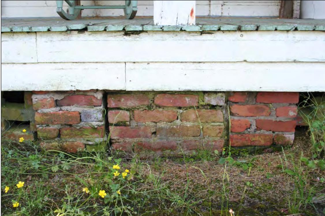
Figure 64. Brick piers supporting the porch of Structure 39-00837. The soft red bricks to the right are likely the original piers. Photograph taken 8 May 2013, facing south.
