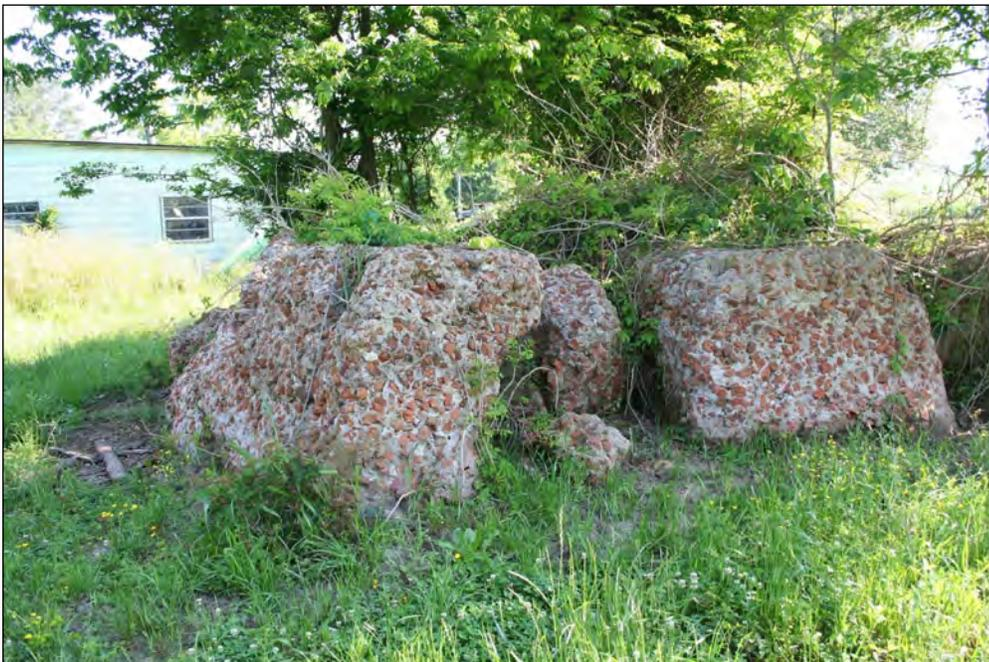
**Figure 67.** Close-up view of Structure 39-00838, from the south. The machinery base to the left has an arched underside, a typical configuration for a grinder base in a sugar mill. The base at right may be *in situ*. Photograph taken 8 May 2013.
