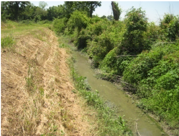
Figure 4.2.2 Bayou Verret Crossing of Route 1
