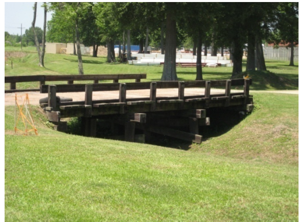
Figure 4.3.2 Bridge over Bayou Verret Route 2
