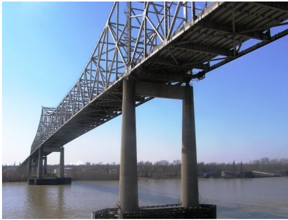
Figure 3.1.3 Sunshine Bridge Ascension Parish, LA
