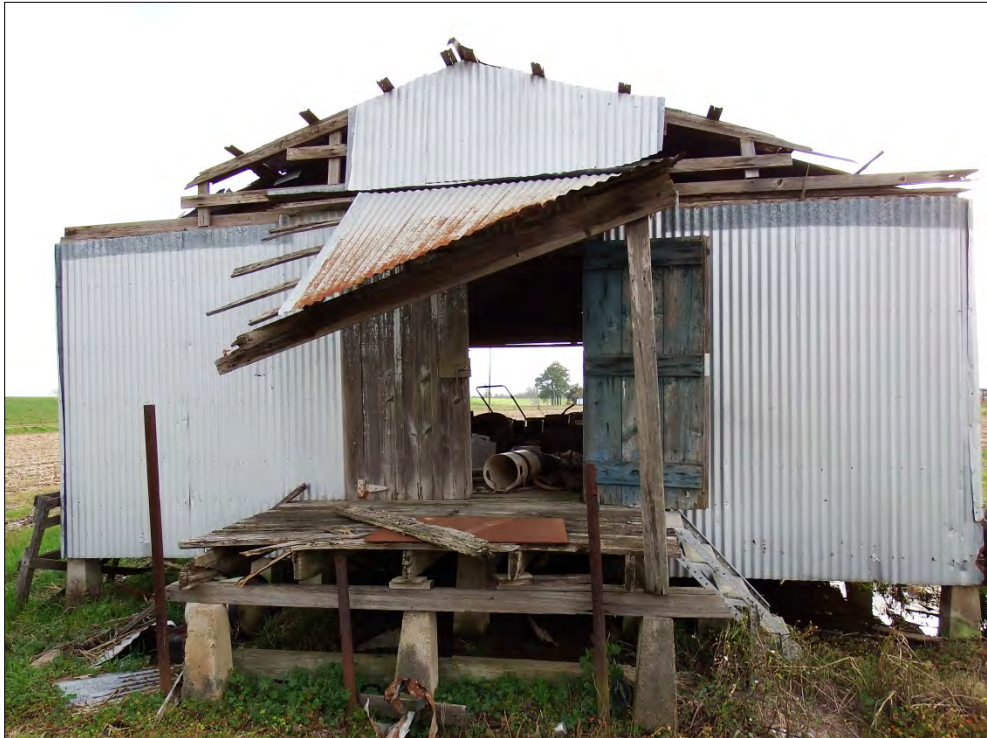
Photograph 2. Shed, Area of Concern, Facing East
