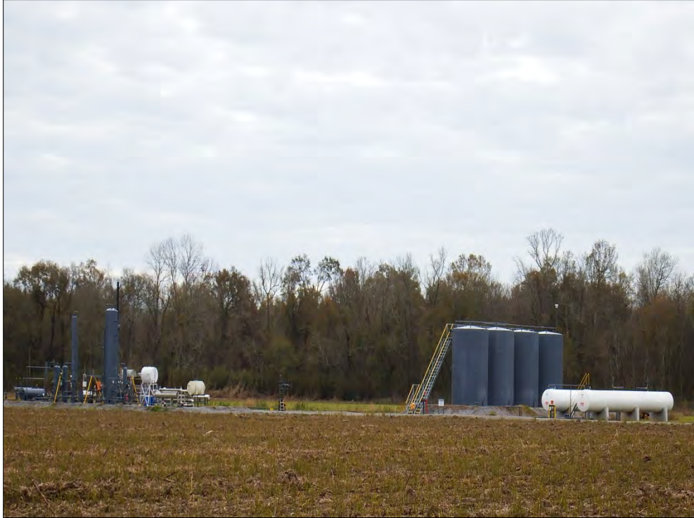
Photograph 23. Active oil Well, Southwestern Corner of Property, Facing Southeast
