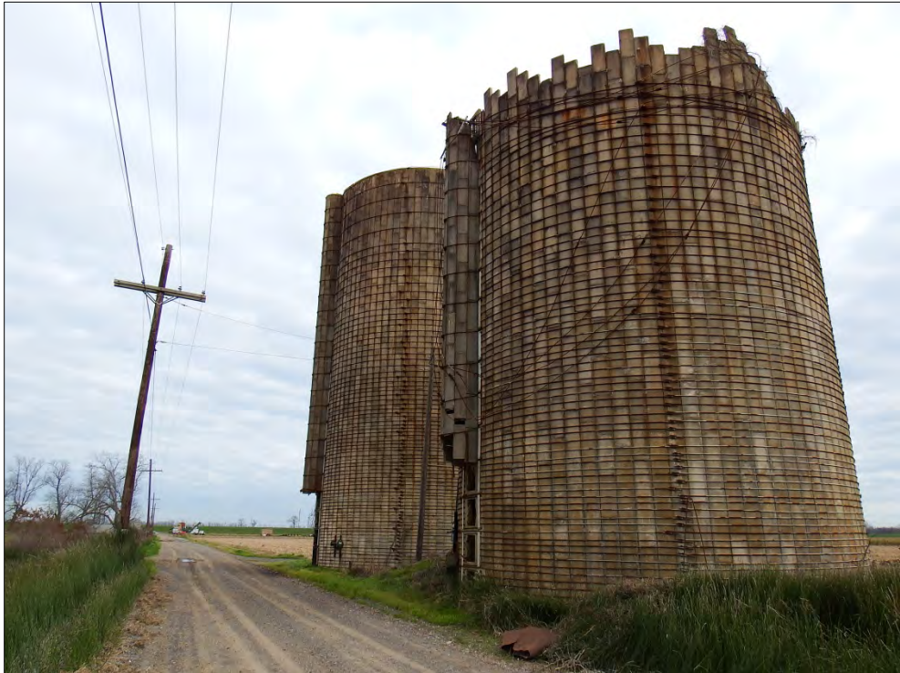
Photograph 14. Grain Silos, Northern Portion of Property, Facing North
