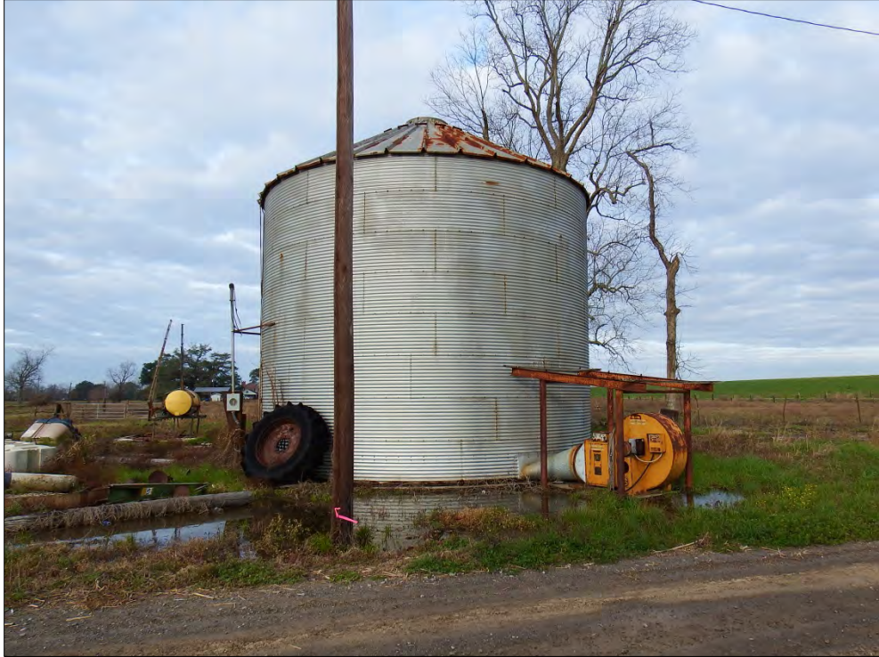
Photograph 1. Grain Silo, Area of Concern, Facing Northwest
