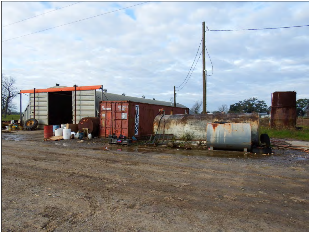
Photograph 6. Quonset Hut, Shipping Container, Stack of Car Batteries, Three Aboveground Storage Tanks, Area of Concern, Facing Southwest
