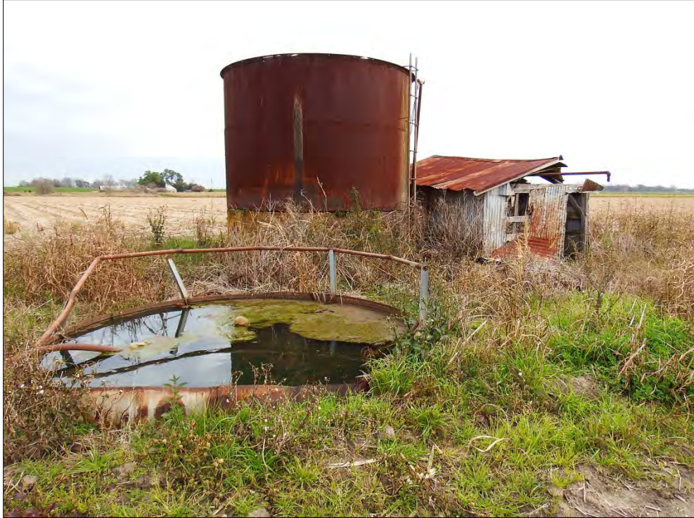
Photograph 13. Well, Pump House, Cistern Northern Portion of Property, Facing Northeast
