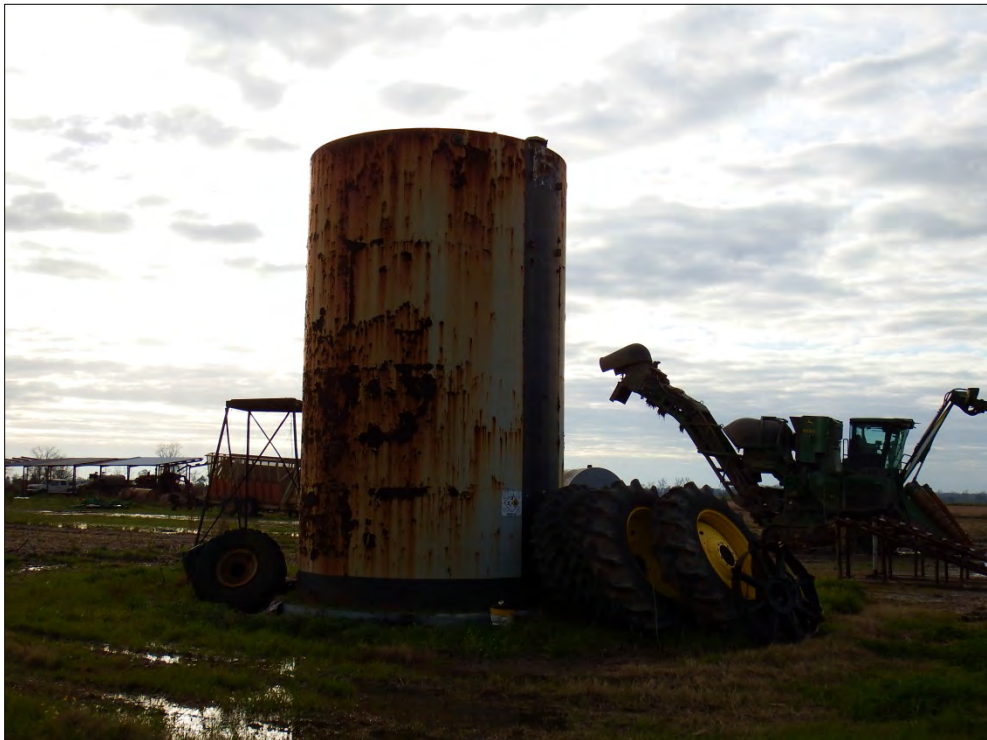
Photograph 4. Aboveground Storage Tank, Area of Concern, Facing East
