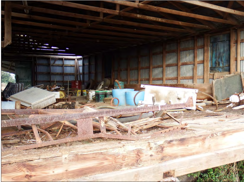
Photograph 3. Shed Interior, Area of Concern, Facing West
