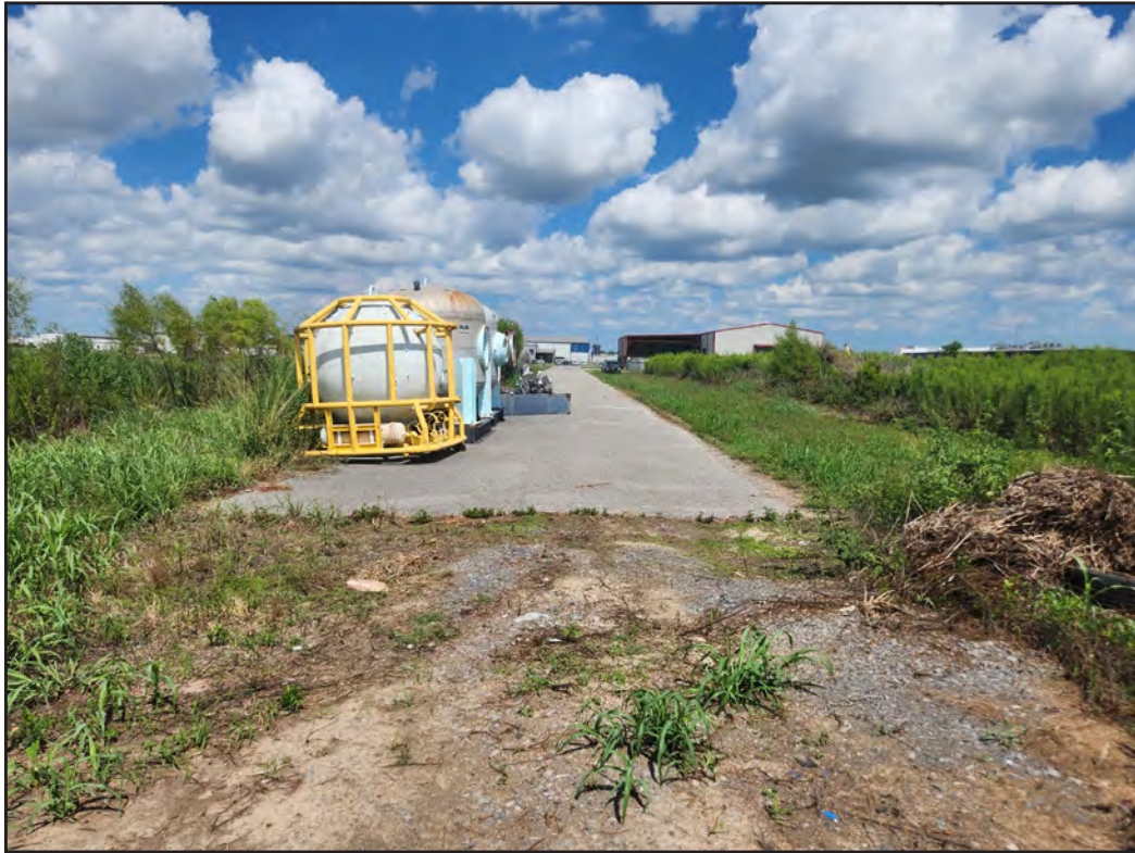
Figure 5.10. View of the access road on the west side of the project area, facing north.
