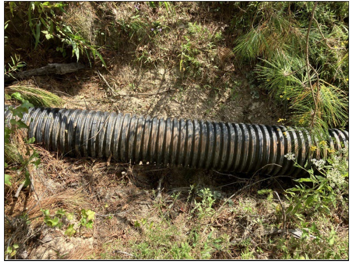
20. Corrugated plastic drainpipe
