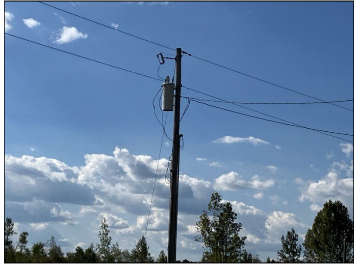
14. Pole-mounted transformer
