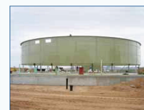
Synchronized jacks are used to erect bolted-panel tanks from the ground up. Workers stay on the ground and perform no hot work which makes tank construction safer compared to field-welded methods.
