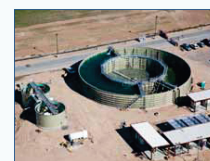
The completed plant is filled and commissioned.
