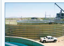
Mechanical components are installed, including blowers, pumps, aeration units, clarifiers, SBR components (when appropriate), grating and plumbing.
