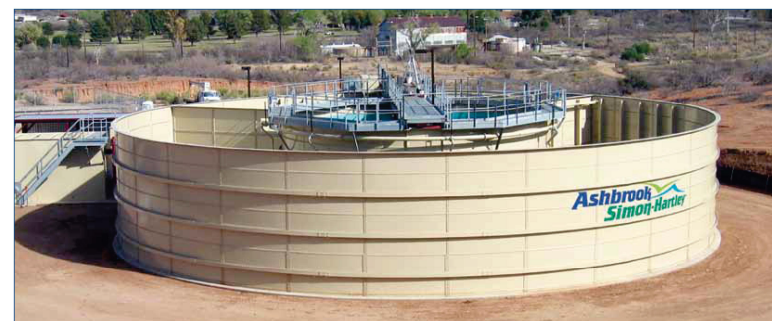
Scope includes: blowers; Wilfley Weber aeration systems; process and clarification tanks; grating, handrails & staircase; pumps and plumbing.
