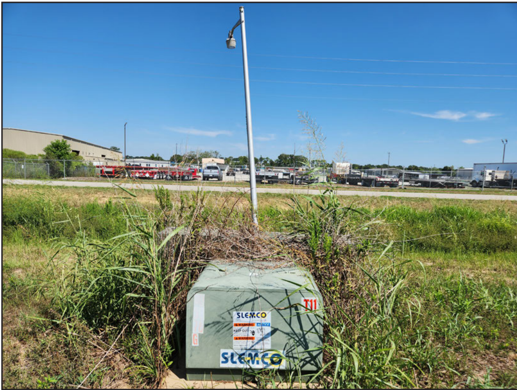
Figure 5.9. View of the streetlight and electrical box on the northern boundary, facing north.
