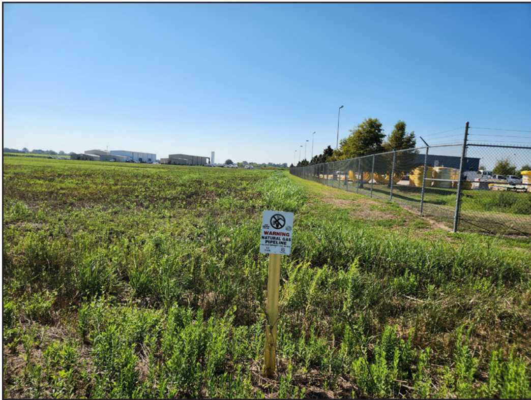
Figure 5.7. View of the pipeline through the center of the project area, facing south.
