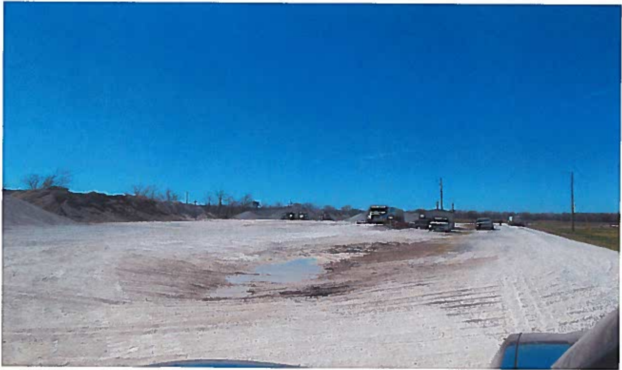
Rock Yard staging site on the subject property
