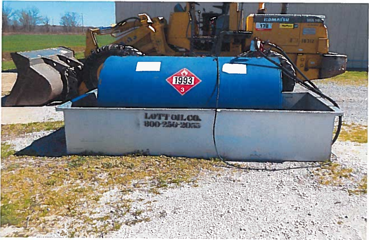
Diesel fuel tank and containment tub located near the entrance to the warehouse
