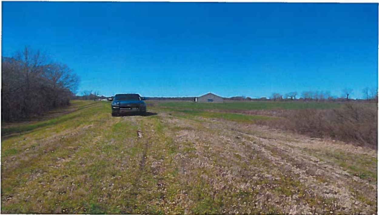
Looking Westerly along the levee near the southeast corner
