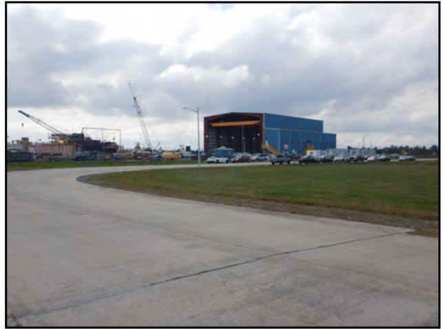
Photo 62: View of the industrial property adjacent to the west-southwest.
