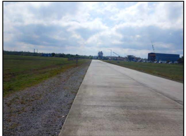
Photo 4: View of Rome Woodard Street, facing south.
