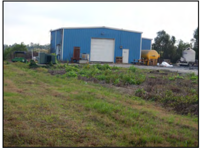
Photo 58: View of a structure, pad mounted transformer, and two additional aboveground storage tanks observed on the property adjacent to the west-southwest of the Subject Property.
