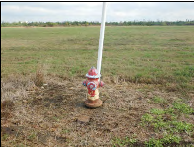
Photo 47: Fire hydrant and water utility vault observed on the northwestern boundary of the Subject Property.
