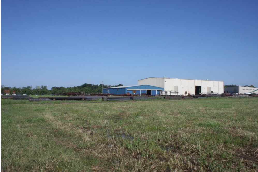
Photograph 1. Smith Tank and Steel Located West of Property
