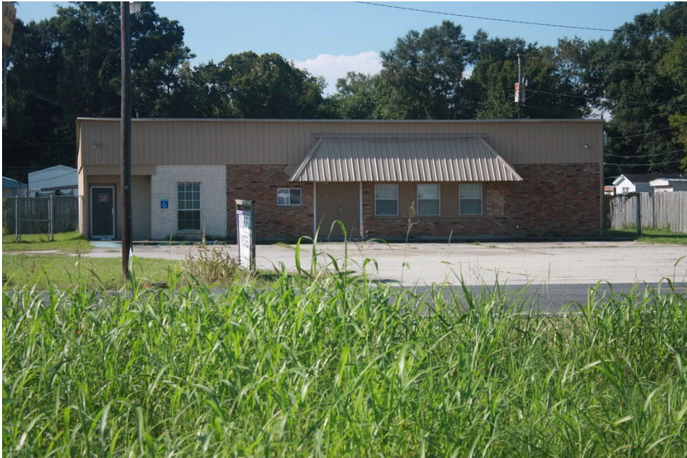
Photograph 16. Closed Oak Village Store Located across Hwy 30 South of Property
