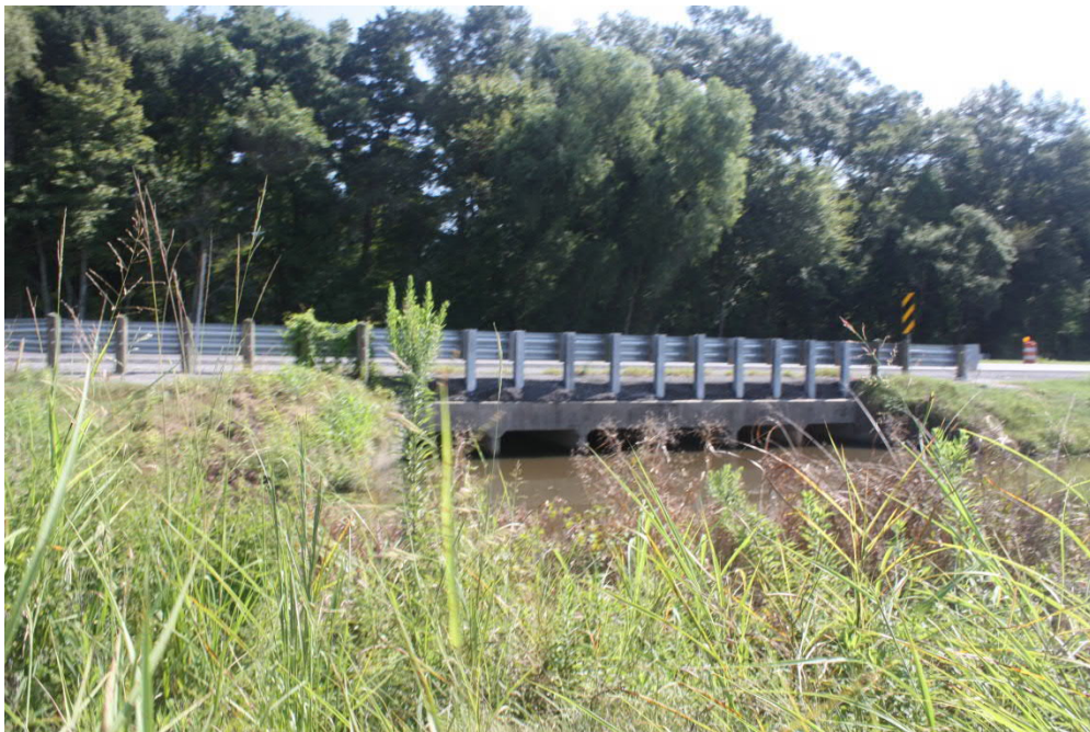
Photograph 24. Eastern Tract Ditch at Airline Hwy
