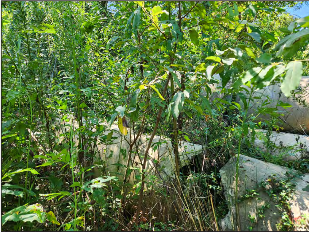
Figure 5.8. View of concrete piping abandoned in the treeline in the western portion of the project area, facing southwest.
