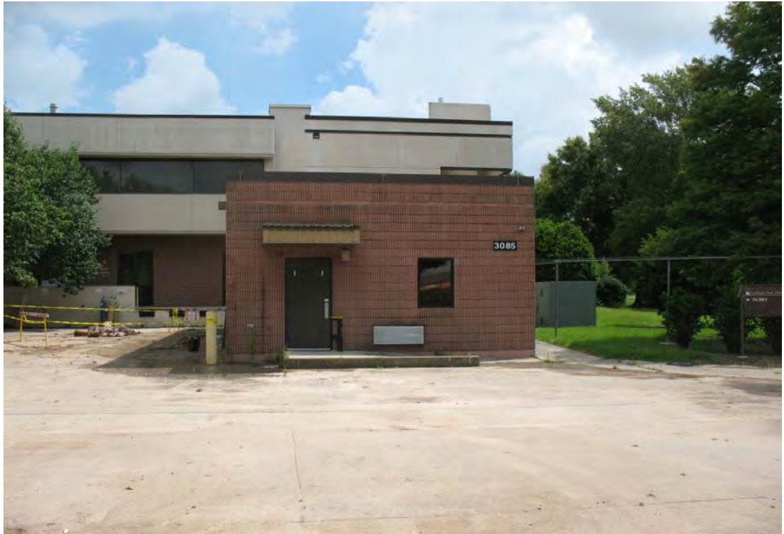
20. Looking north at Buildings 3085 and 3100.
