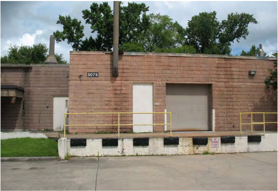
19. Looking north at Building 3075.
