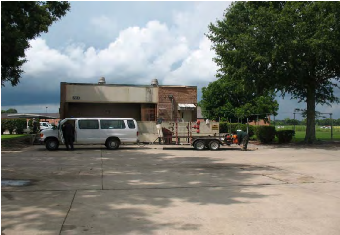
21. Looking south at Building 3055.
