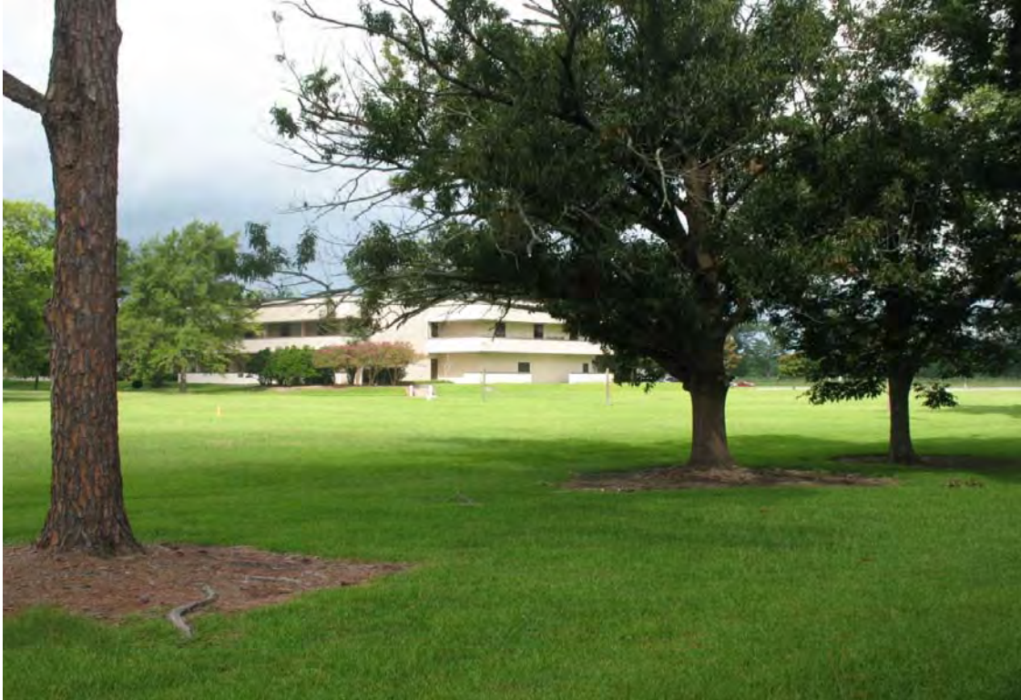
18. Looking southwest at Building 3100.
