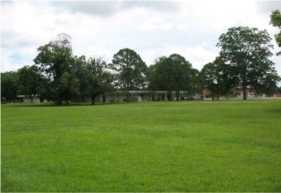
15. Looking northeast at Building 3005 and Building 3010.
