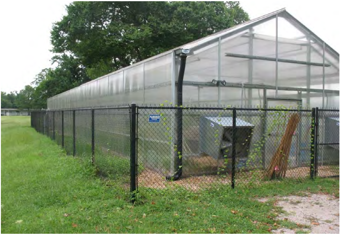
23. Looking north at the greenhouse (Building 3015).
