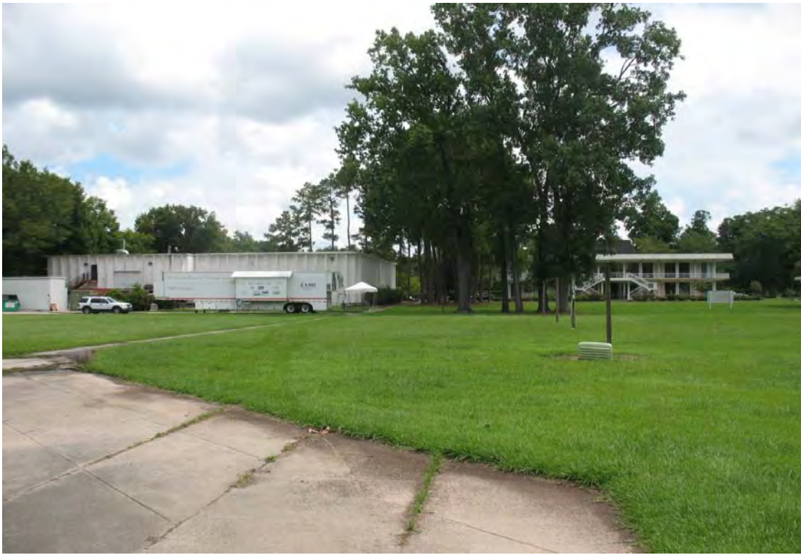
17. Looking north at Building 3000 and Building 3110.
