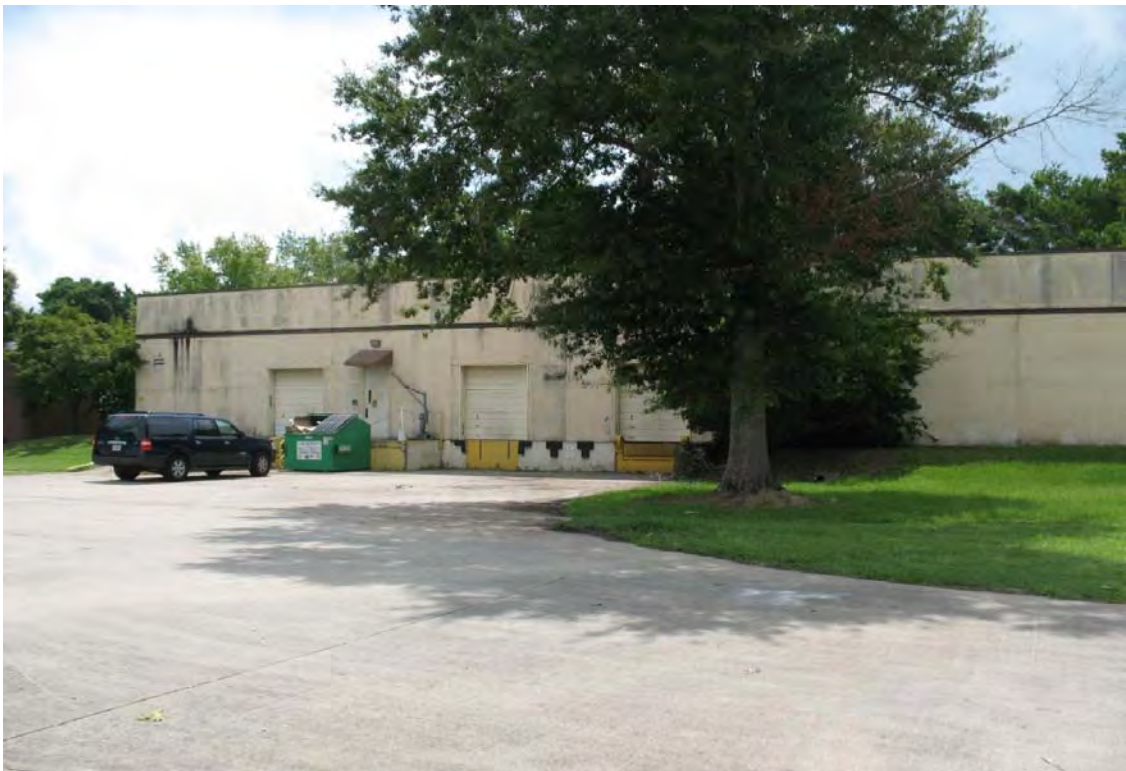
24. Looking east at Building 3030.
