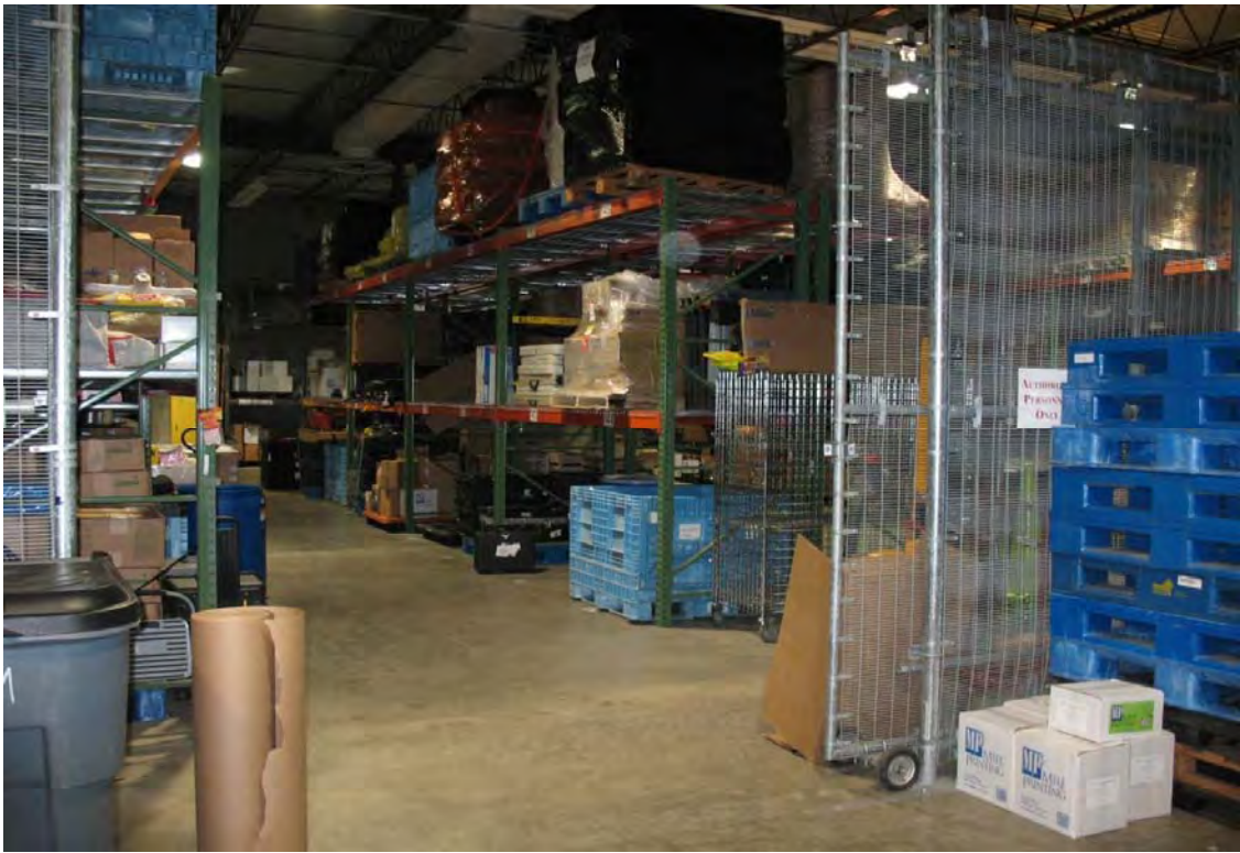
37. View of the interior warehouse space located in Building 3030.
