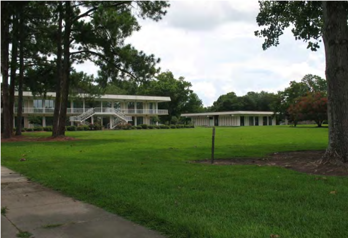
16. Looking north at Building 3000 and Building 3005.
