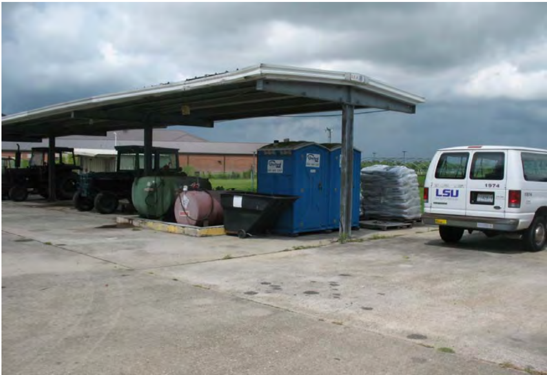
26. Looking southwest at Building 3045.
