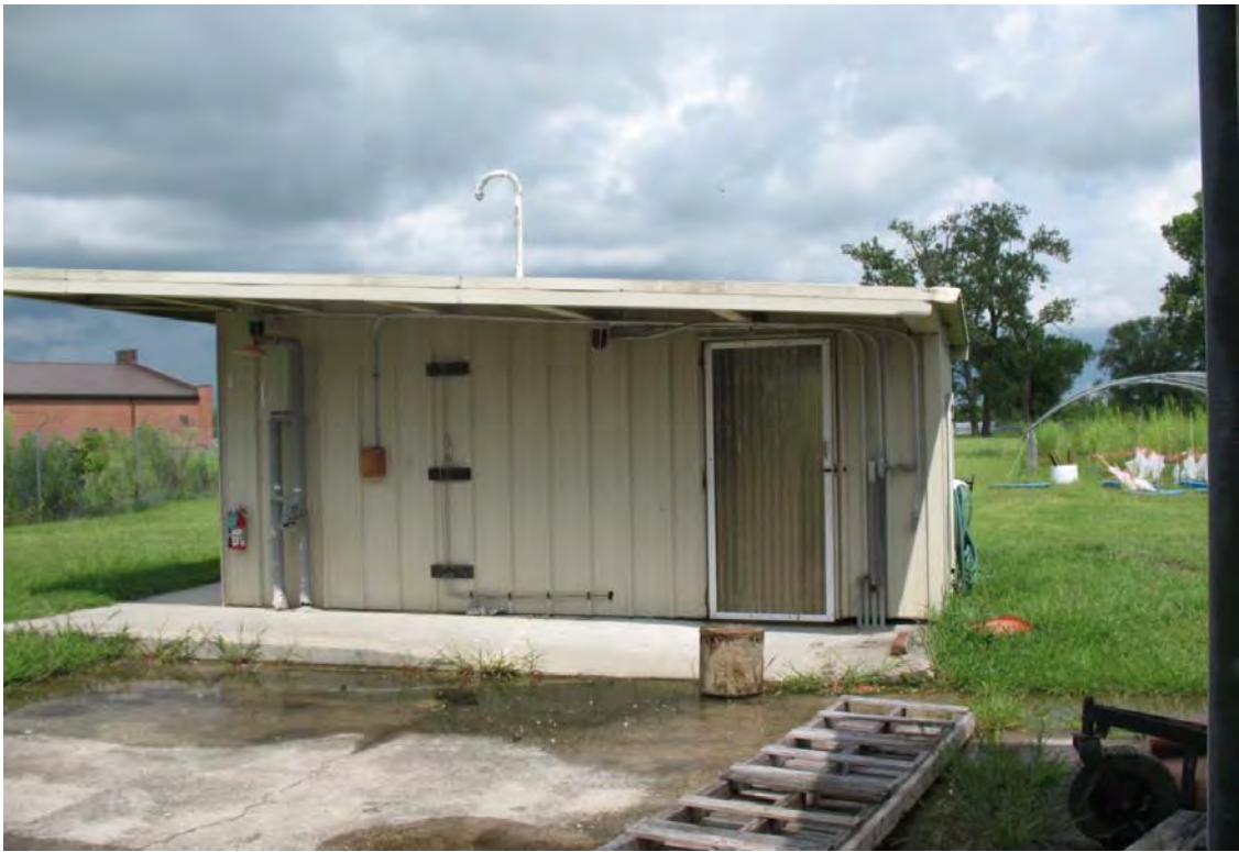
25. Looking west at Building 3070.
