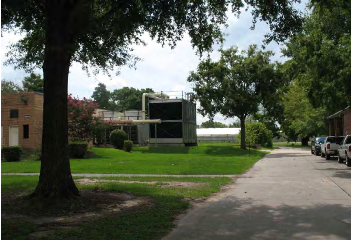
22. Looking east at Building 3025 and the cooling tower associated with Building 3020.
