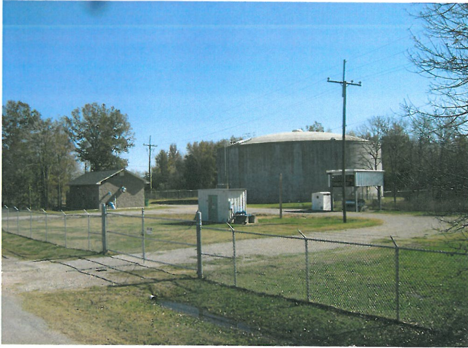
NEW GROUND WELLS AND GROUND STORAGE TANK CONSTRUCTED IN THE EPPS FIELD IN 2010 FOR CONAGRA
