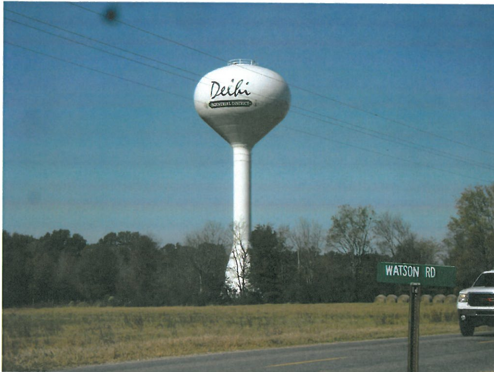
NEW 750,000 GALLON ELEVATED STORAGE TANK CONSTRUCTED AT THE CONAGRA PLANT IN 2010
