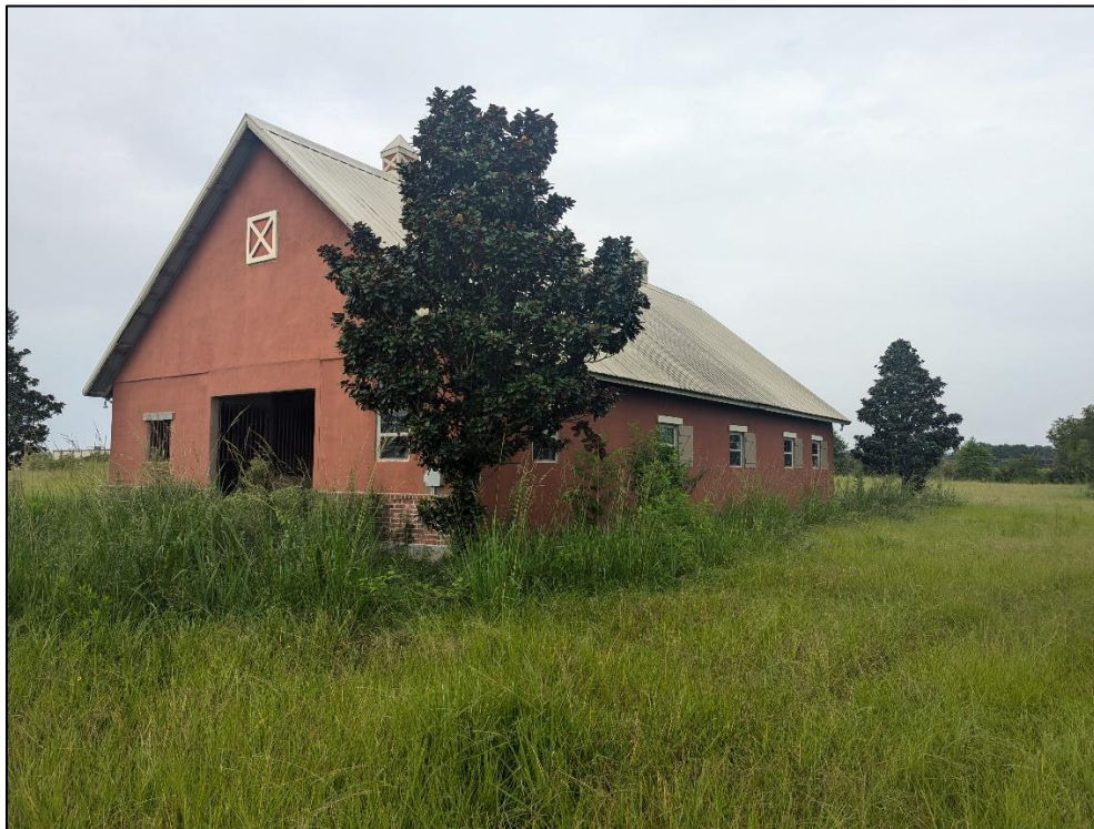
Figure 21. Modern barn within direct APE, facing southeast.
