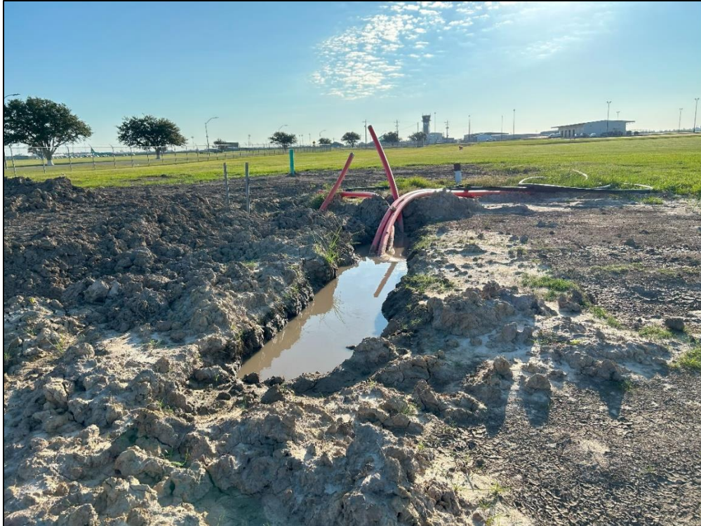
Figure 18. Construction within the southern portion of the direct APE.
