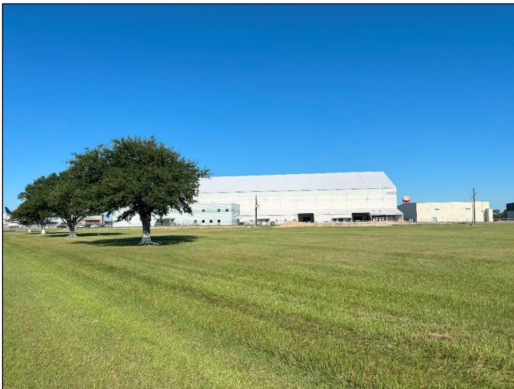
Figure 19. Structures within the northern portion of the direct APE, facing west.
