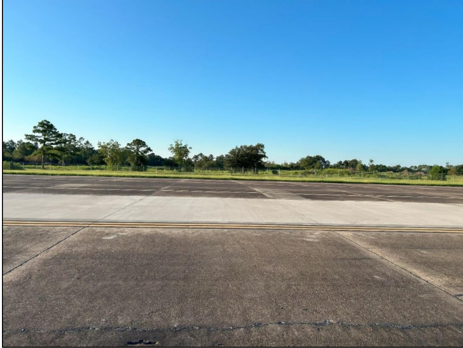
Figure 16. Concrete in the southern portion of the direct APE, facing south.
