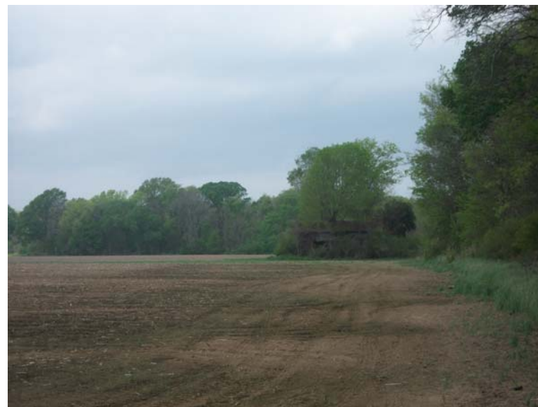
View of building along the northern edge of the site.
