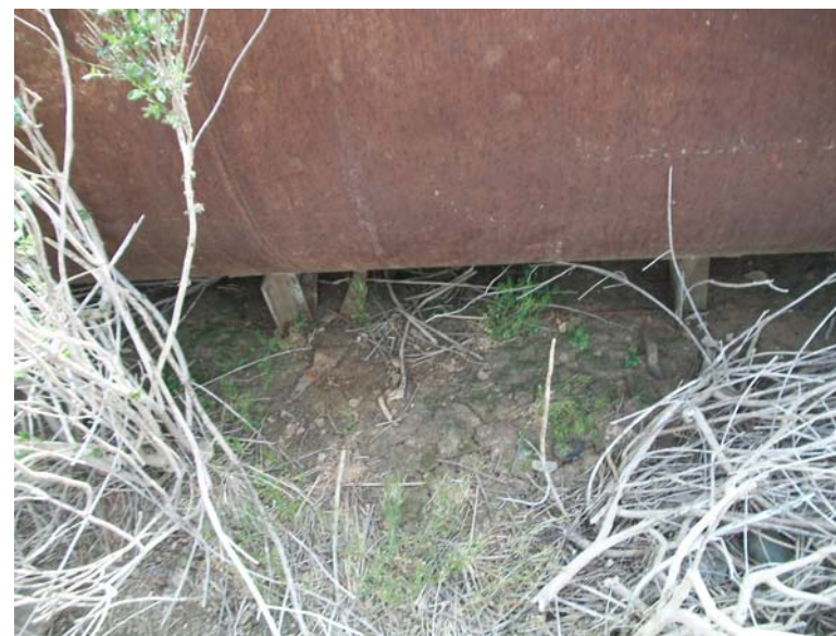
Soil below the AST.
