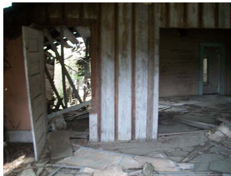
View of the interior of the building.
