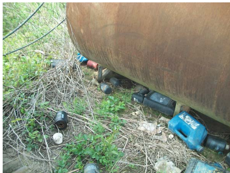
View of waste oil filters and empty oil containers below the AST.
