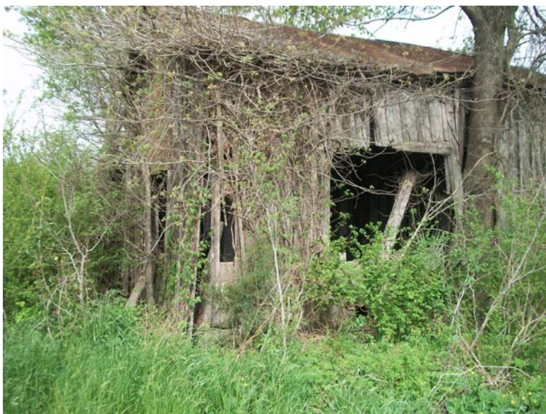
View of east side of the building.
