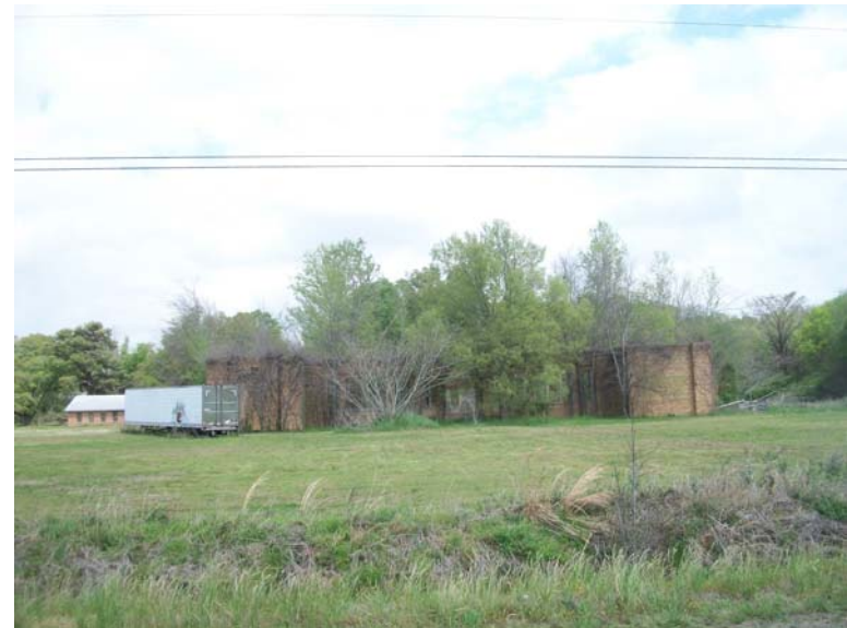
View of vacant building on adjoining property to the north.
