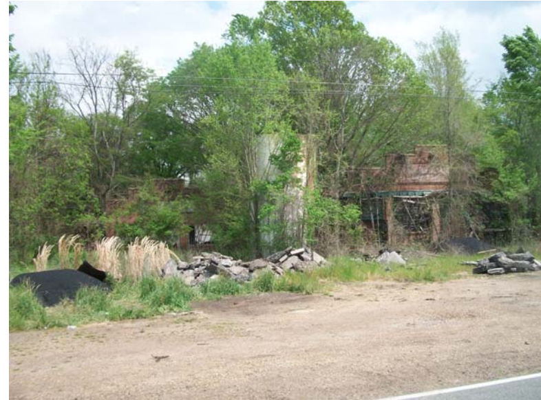
View of abandoned buildings, construction debris, and AST north of Hwy. 80.
