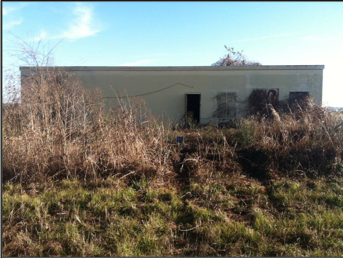
Figure 6.14. Building 2 overview, view east.
