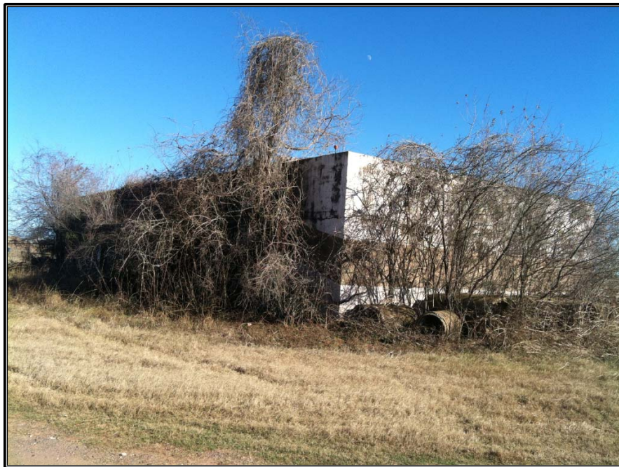
Figure 6.16. Building 4 overview, view east.
