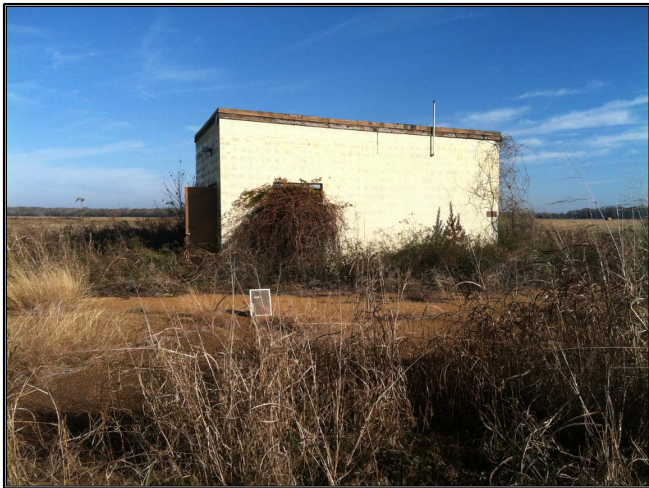
Figure 6.15. Building 3 overview, view north.
