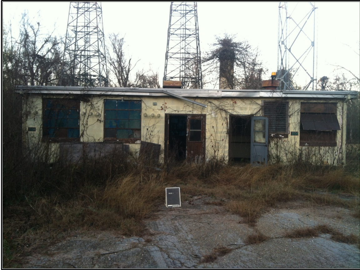
Figure 6.13. Building 1 overview, view west.
