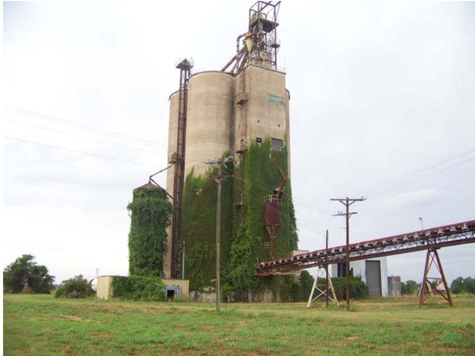
**Photograph 1. Grain silo, showing flammable shed, shop, dryer on left, truck dump on right, and conveyor**
