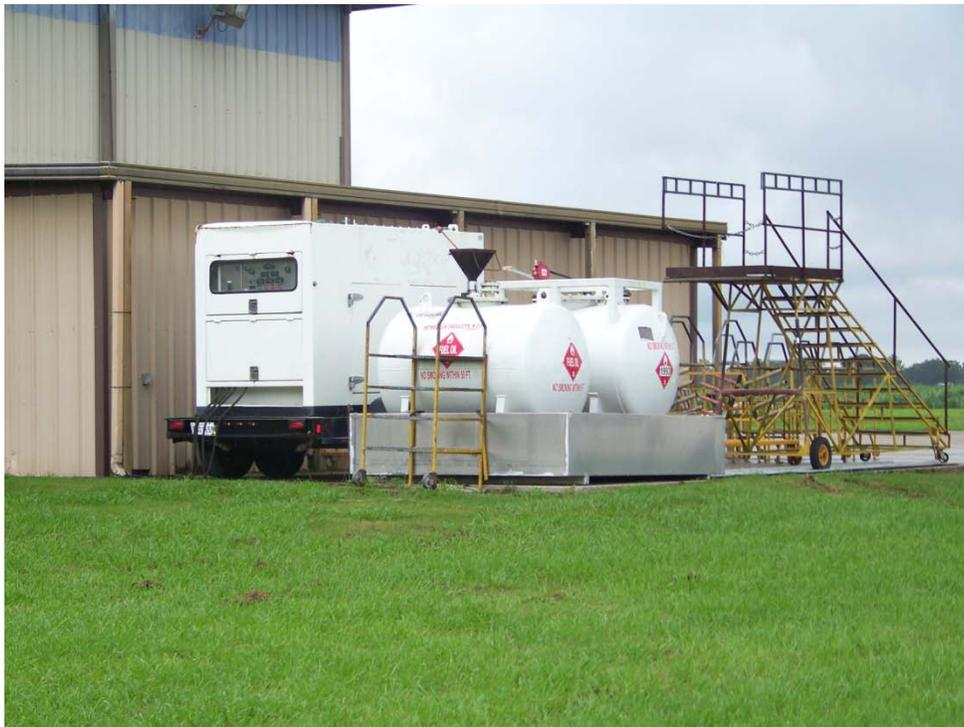
Photograph 6. Diesel and waste oil ASTs at heliport
