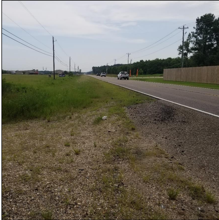
Figure 13. From dirt road depicting S. Frost Rd, facing north.
