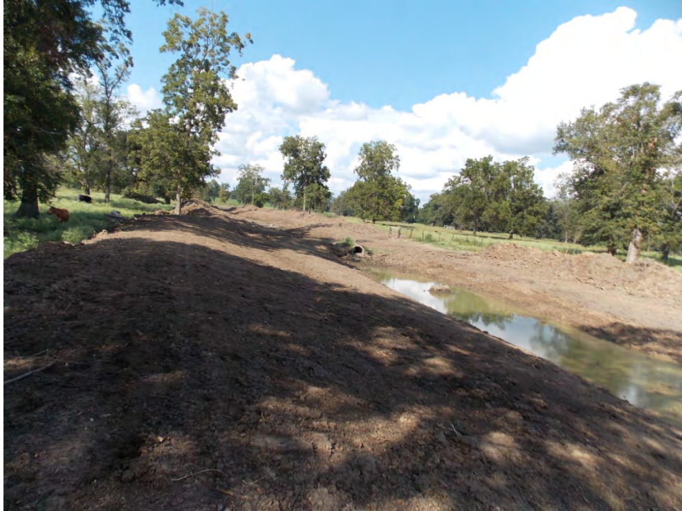
Photograph 7. Drain Improvement Associated with Relief Wells, Facing North
