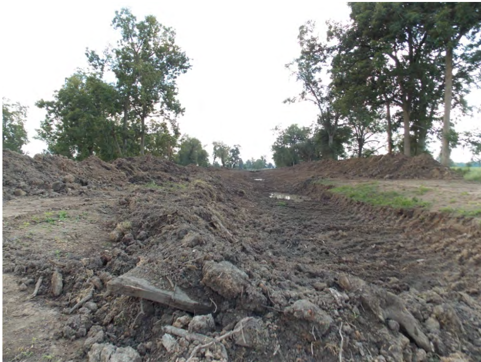
Photograph 6. Drain Improvement Associated with Relief Wells, Facing South
