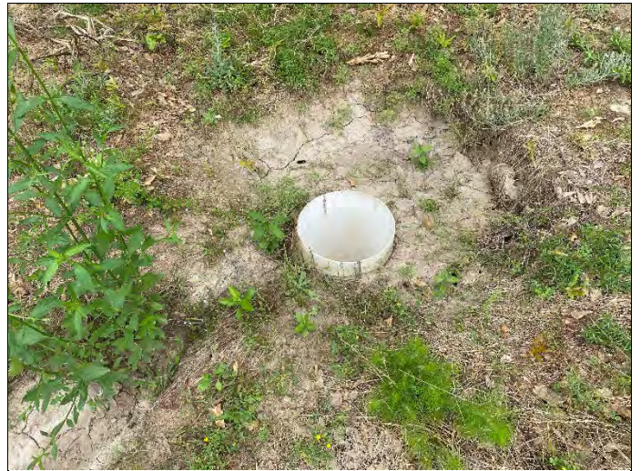
4. Typical field drain installed along the western edge of the site
